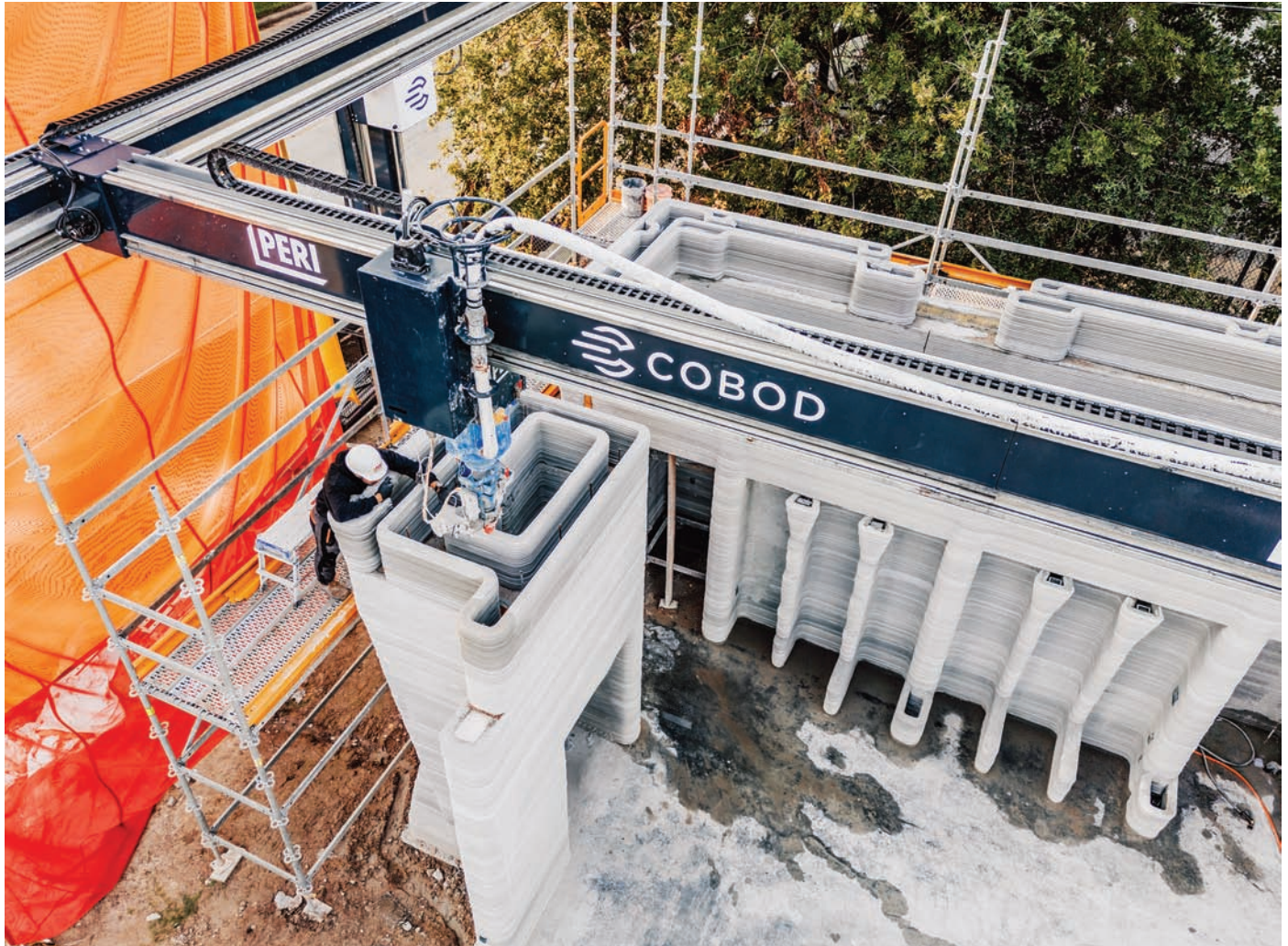
FIG. 2. 3D printer gantry system printing a wall section. Source: https://weprinthomes.com/ .
