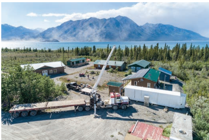
FIG. 1. Installation of the Cropbox at the Kluane Research Station.
