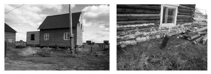
FIG. 5. Two methods of protecting permafrost: (left) by creating an insulating layer under new house construction and (right) by retrofitting existing buildings. Churapcha region, Central Yakutia (photos by A.N. Fedorov and P.P. Federov).
