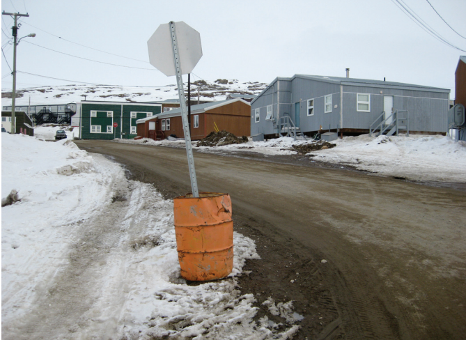
FIG. 4. This photo of a stop sign anchored into place with an old oil drum demonstrates the recycling of old products. Many of the street signs in the Arctic can't be placed into the ground because of the permafrost. Anchoring the signs with old oil drums filled with rocks has been an innovative way to meet needs and re-use old materials.
