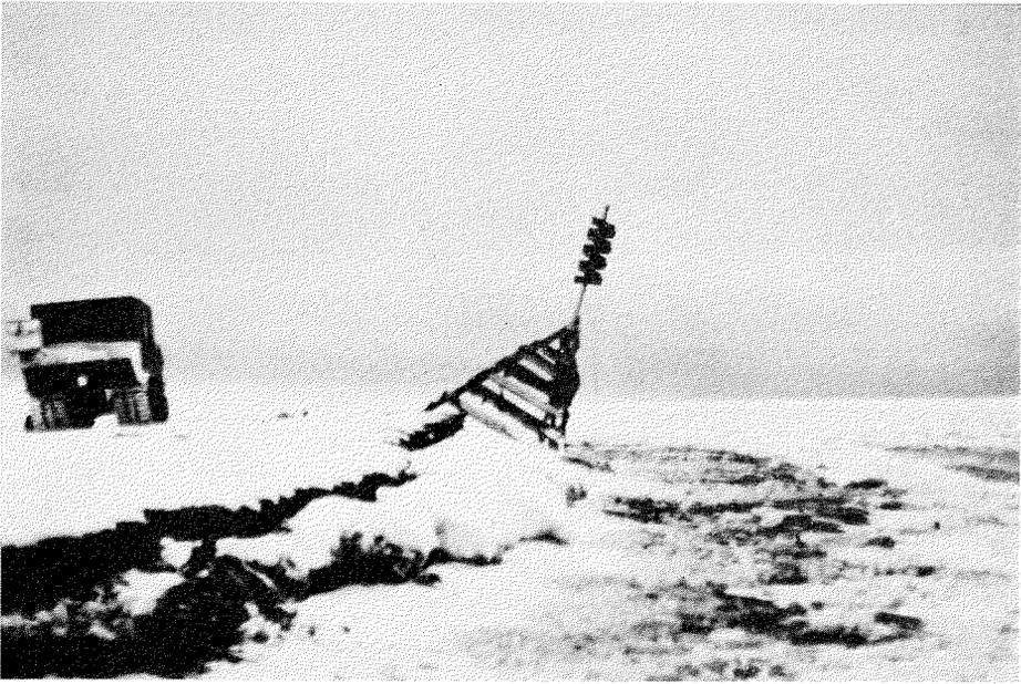
**Fig. 2.** Triangulation station 'Doctor', at the extreme end of the sand spit projecting southeast from Point Barrow, being undermined by wave action. 20 October 1949. This station was recorded as being 85 feet from the shoreline in September 1945.
