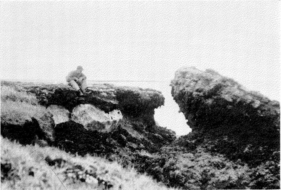
Fig. 5. Breakdown of bluff along ice wedges near triangulation station 'Goon'. Note ice exposed just beneath the seated figure.
