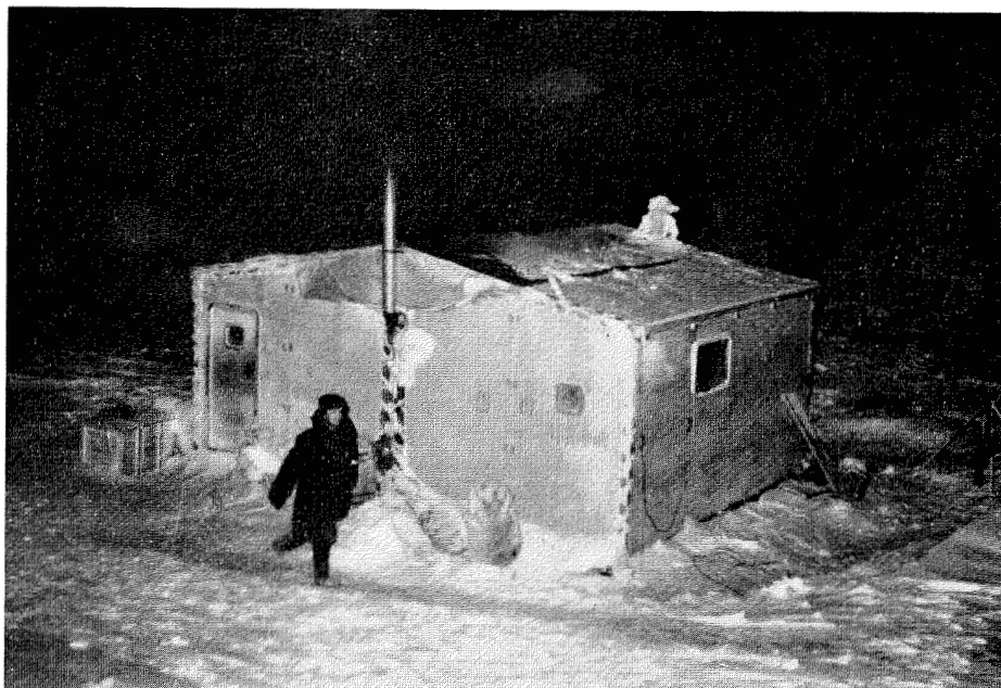
Fig. 4. Two prefabricated huts at North Pole 3, which have been joined together, autumn 1954.
