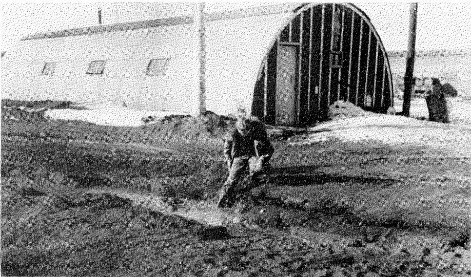
Fig. 4. Slump in the gravel street at the U.S. Navy camp near Barrow along a heated sewage line. The thaw penetrated more than 7 feet and the surface dropped more than 2 feet in 2 years. May 17, 1950.
