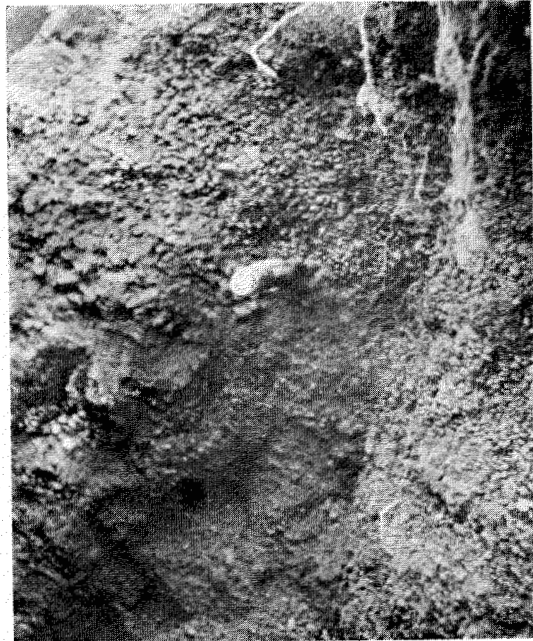
Fig. 8. Gravel exposed in trench at the base of a residual-slope feature.
