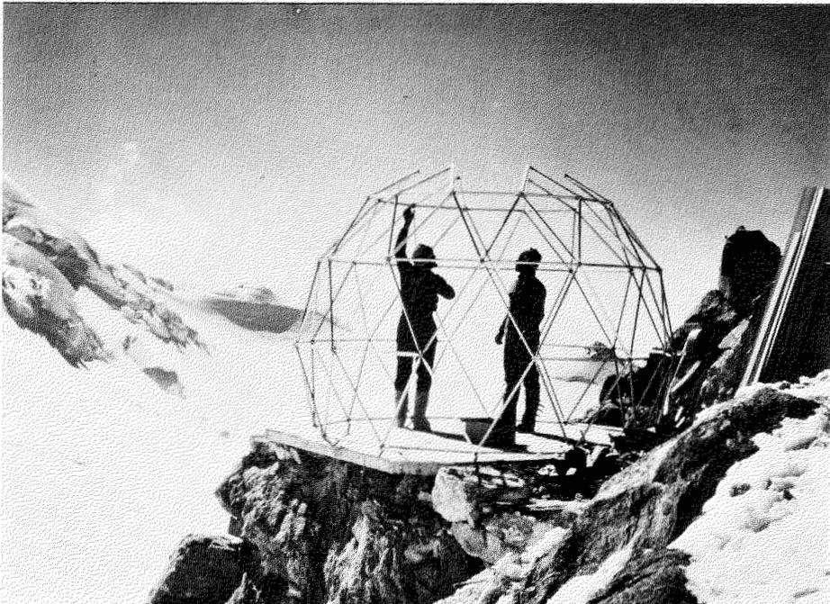
FIG. 3. Partly completed frame showing elemental structure. The NW Col is to the left. (Photo by J. Wyss).
