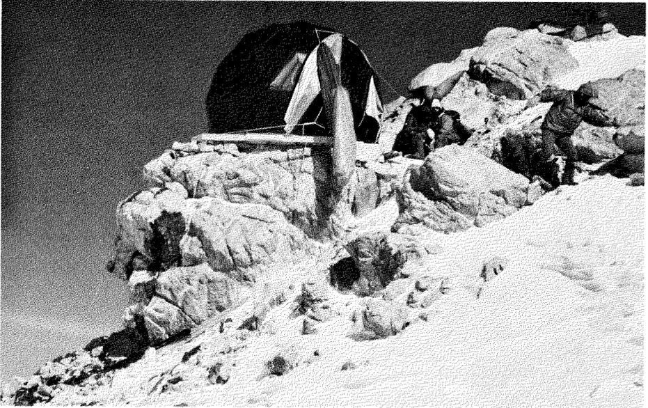
FIG. 4. Completed hut showing part of outer canopy peeled back over inner nylon cover. (G. Holdsworth).
