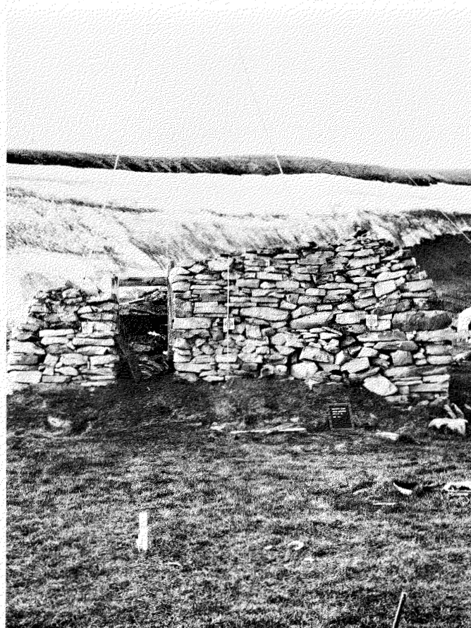
FIG. 15. A photographic elevation of the south wall of Kellett's storehouse, as found in July 1978.
