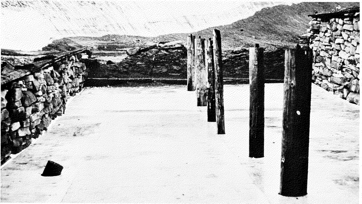
FIG. 12. The insulated floor in place.
