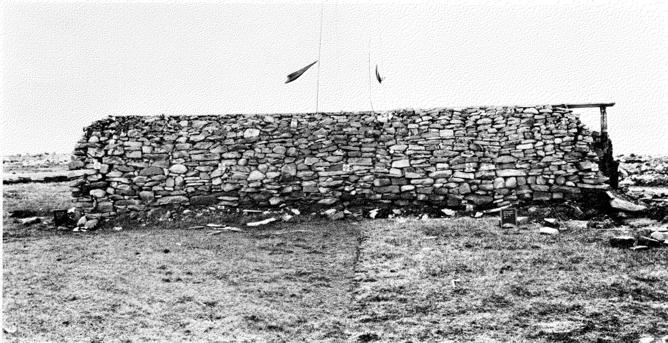
FIG. 14. A photographic elevation of the east wall of Kellett's storehouse, as found in July 1978.
