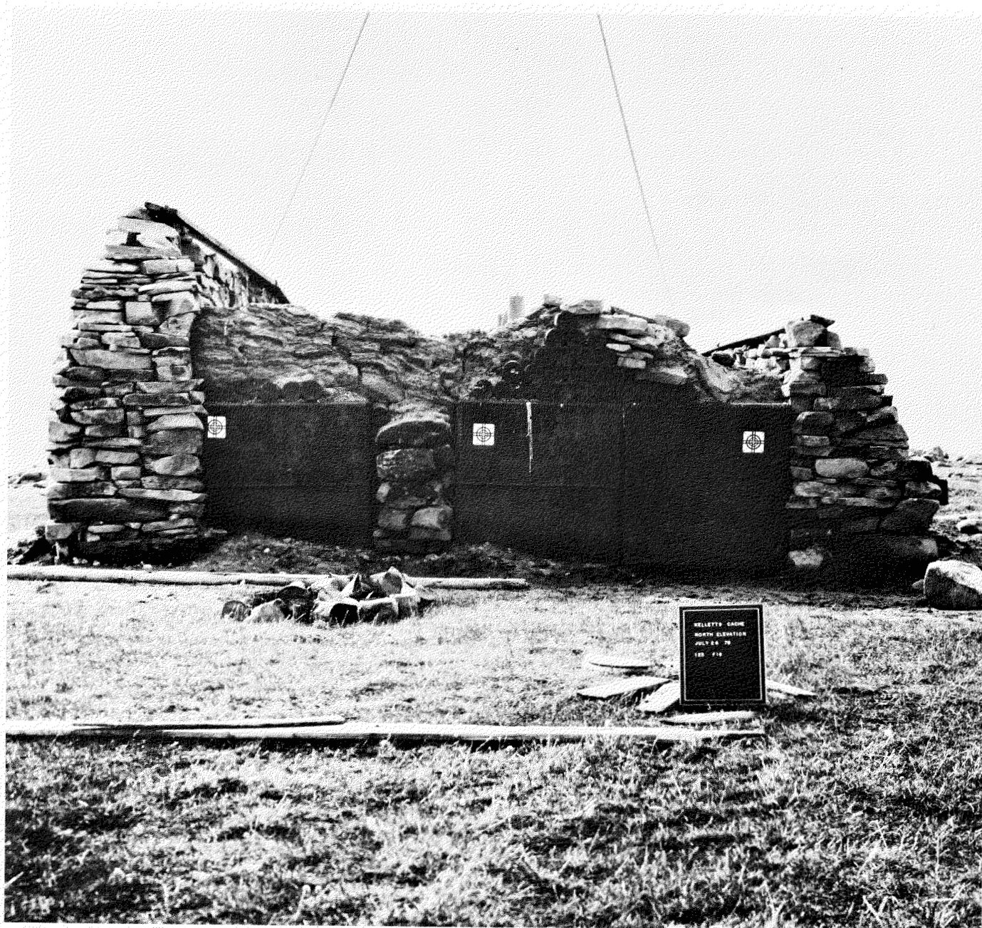
FIG. 10. The north wall of Kellest's storehouse after it was reconstructed.
