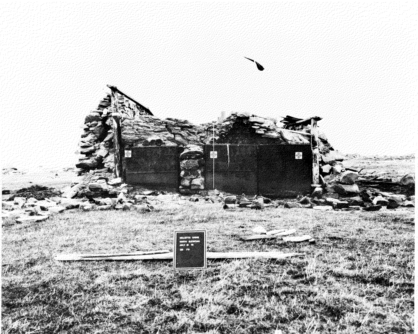
FIG. 6. The north wall of Kellett's storehouse before it was reconstructed. Note the ballast tanks in the lower portion of the wall.
