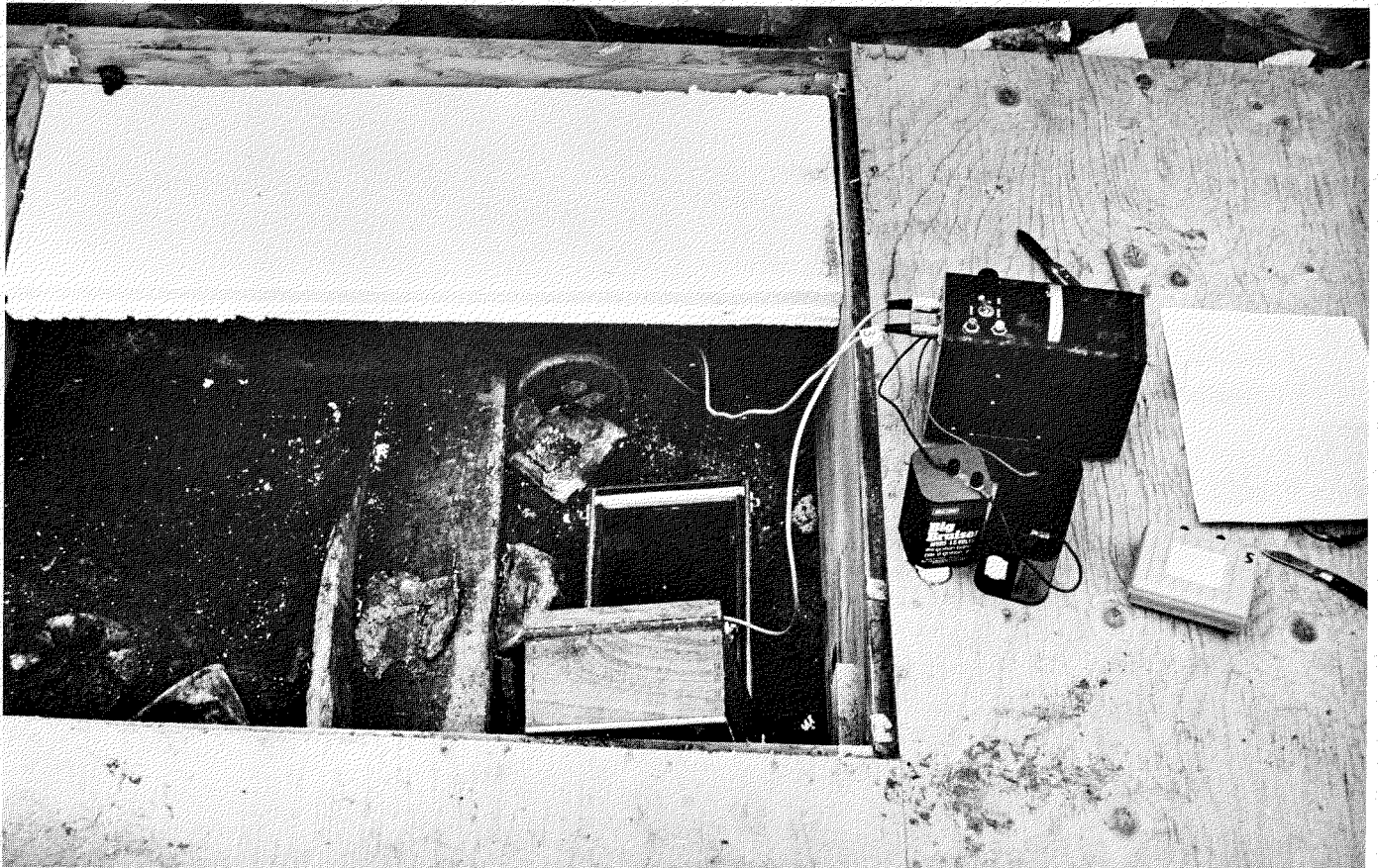
FIG. 13. The installation of the hygrothermograph in a compartment beneath the insulated floor. The wires leading out from the instrument are connected to temperature and humidity sensors.
