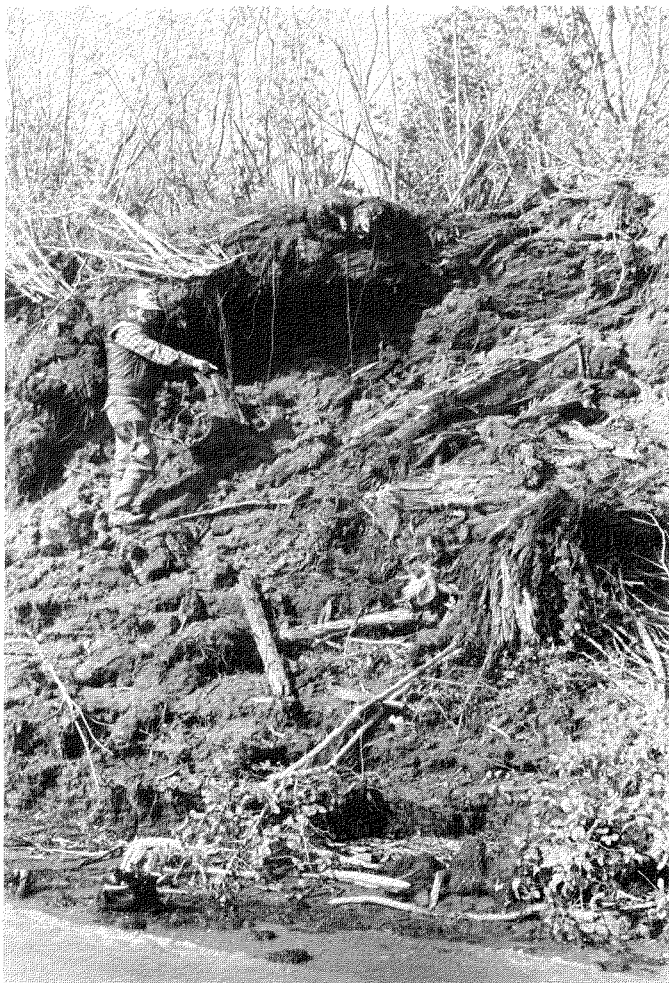
FIG. 2. Collapsed bank at the Bombardier Channel site. Most of the logs that have fallen down the bank are from the burial feature.
